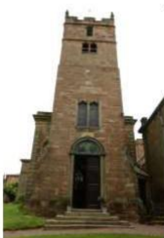
Entrance to St Andrews Church
